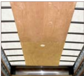
Plywood ceiling runner
